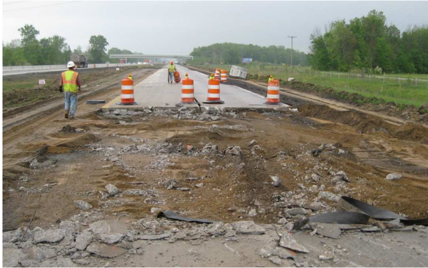
Figure 82. Overview for test bed 2
