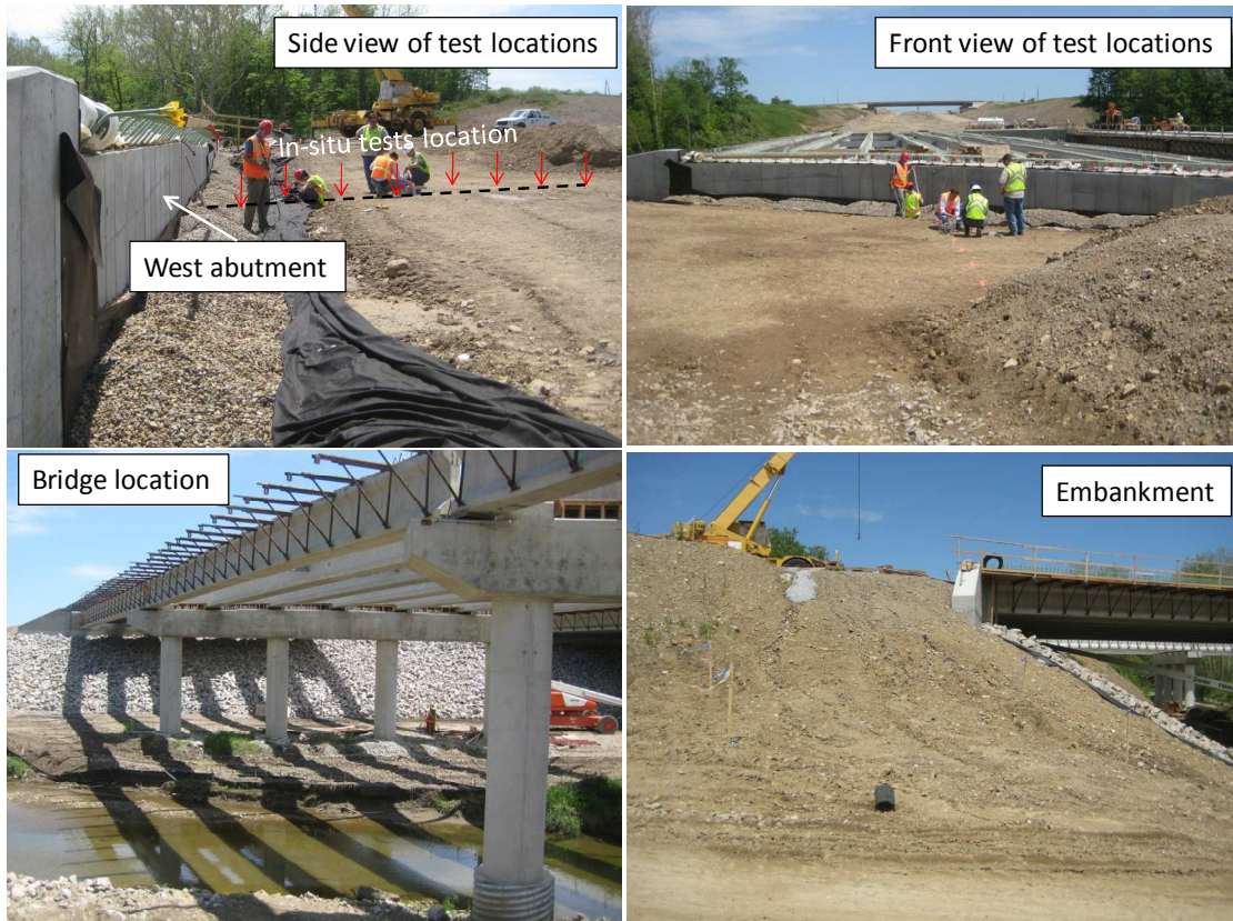
Figure 69. Bridge #5 (LIC-37-1225L) at Licking 161 over Moot Creek
