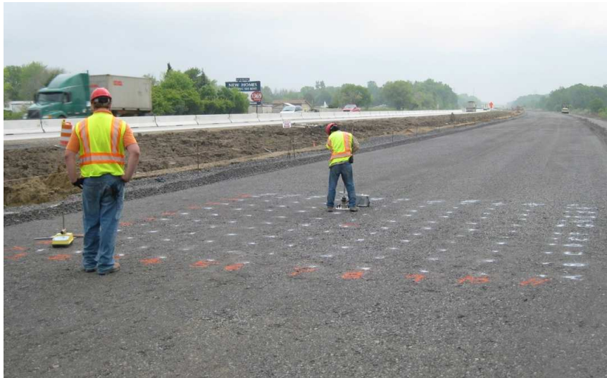
Figure 81. Overview for test bed 1
