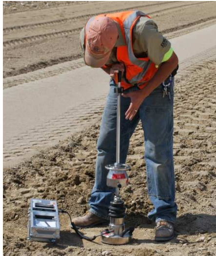
Figure 8. Light weight deflectometer test with 200-mm diameter plate
